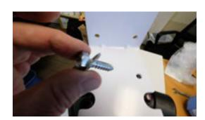
Next mount the filter housing to the wall using appropriate fasteners for your wall material. Mount on a solid surface or secure a board or piece of plywood on wall stud. Filter housing will be heavy when full of water.
